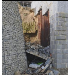
Collapsed Blockwork
