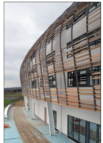
Brise soleil panels
