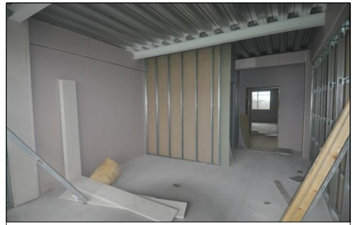
Bedroom during construction May 2014
